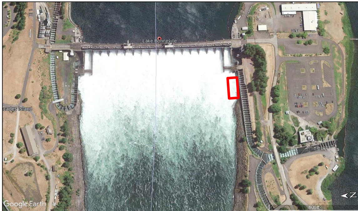
Figure 2 Bonneville Dam Spillway. Red box indicates approx. inspection area.
